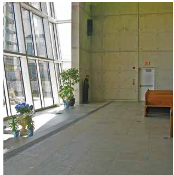
Example of a floor mounted diffuser.
