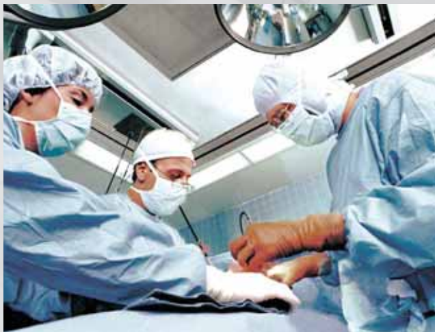
Steri-System Hospital Operating Room Air Distribution System
