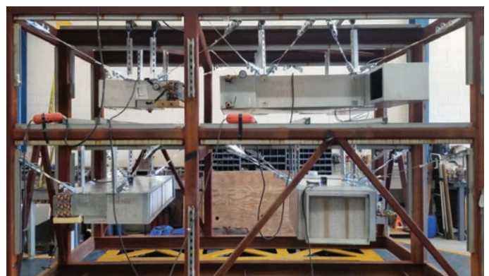
Horizontal Fan Coil Units Shake Table Test
