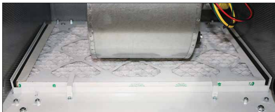
Figure 5. Pre-filter Replacement
