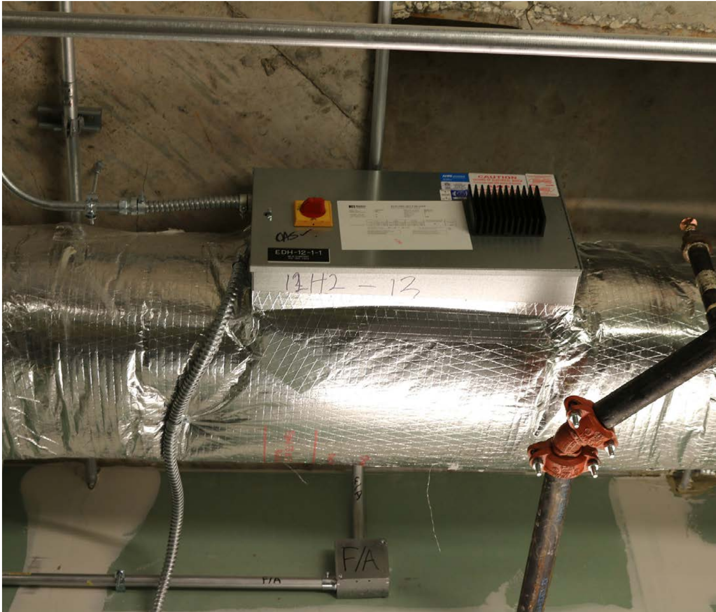
ELECTRIC DUCT HEATER Model: DHRS with optional SCR
